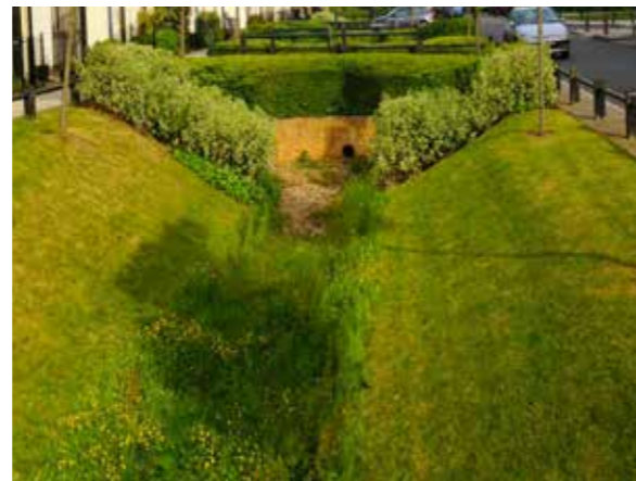
Example of a road side swale
