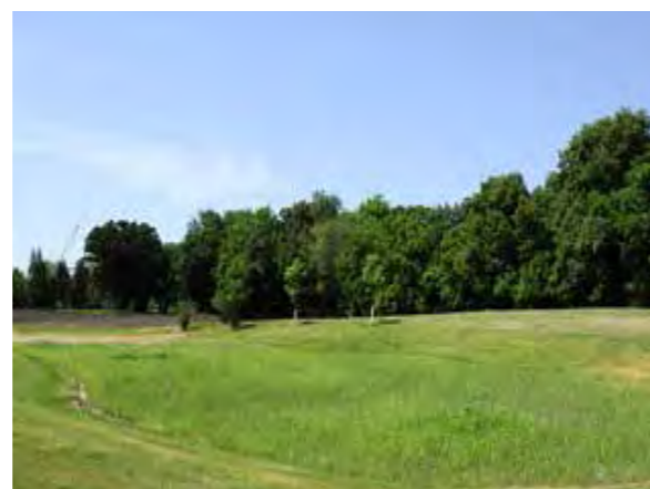
Example of a dry detention basin
