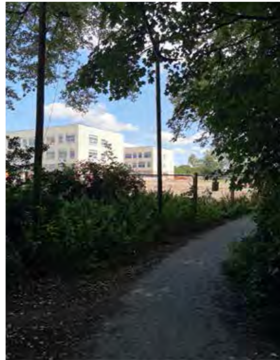
View of the Mildenhall Hub from the Public Right Of Way
