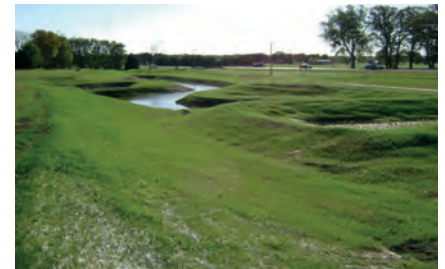
Example of a part wet detention basin
