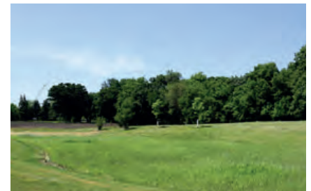
Example of a dry detention basin
