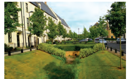
Example of a road side swale
